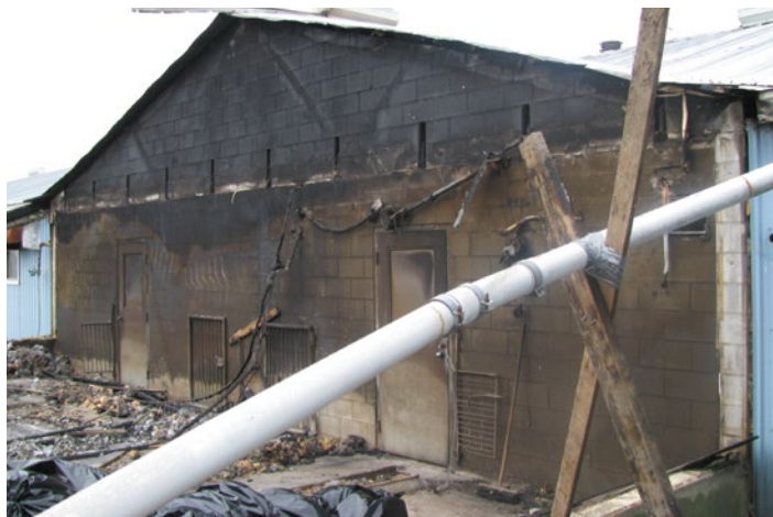
Figure 3.1. Example of a fire separation that served its purpose in a swine complex, preventing the fire from spreading to the rest of the barn.
